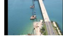
Ayres Associates Courtney Campbell Multiuse Trail Bridge FDOT Distr...
