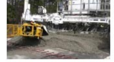
Avcon SR 600 Pavement Rehabilitation FDOT District V
