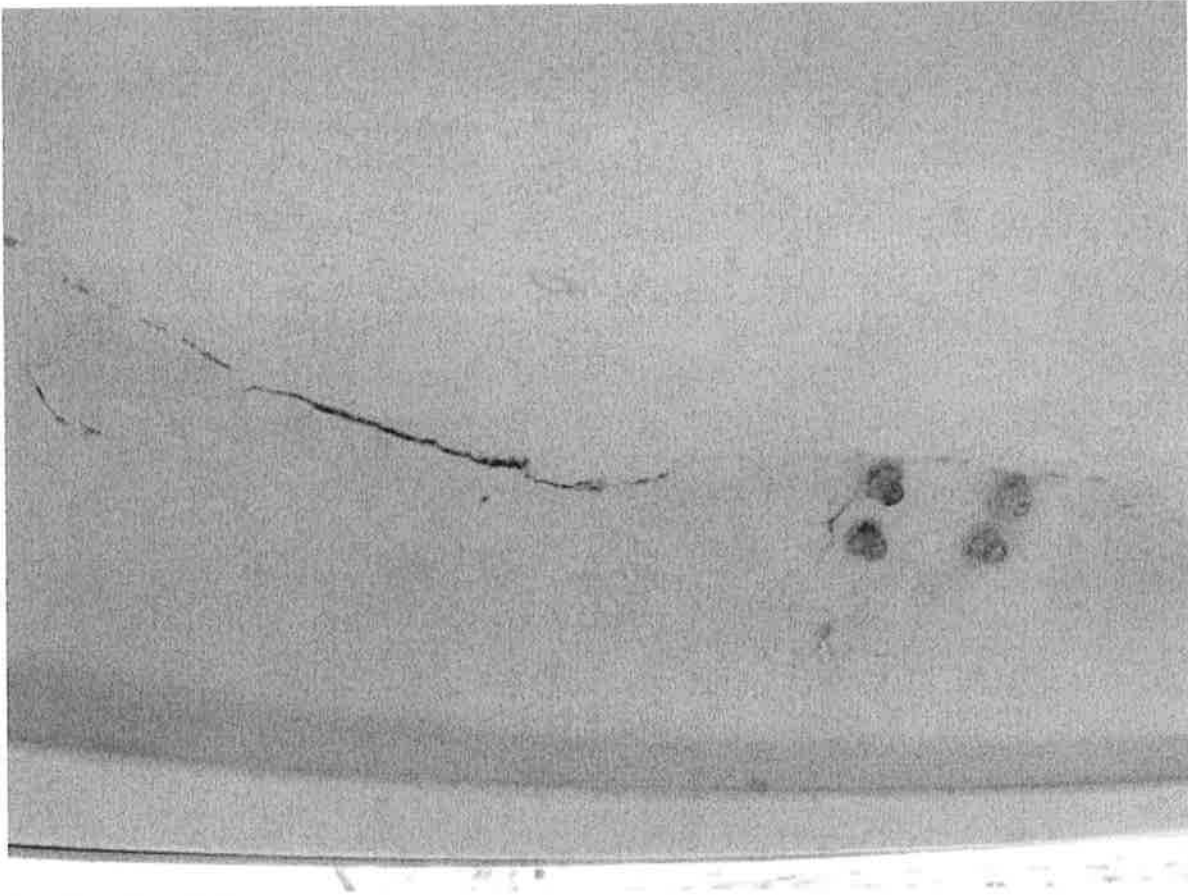
Port side underneath fresh crack
