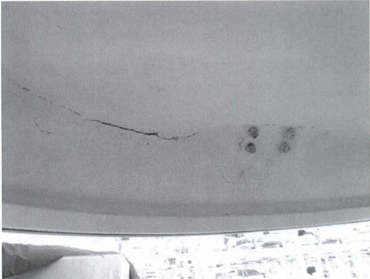
Fresh crack found underneath the swim platform associated with the exterior crack on the port side
