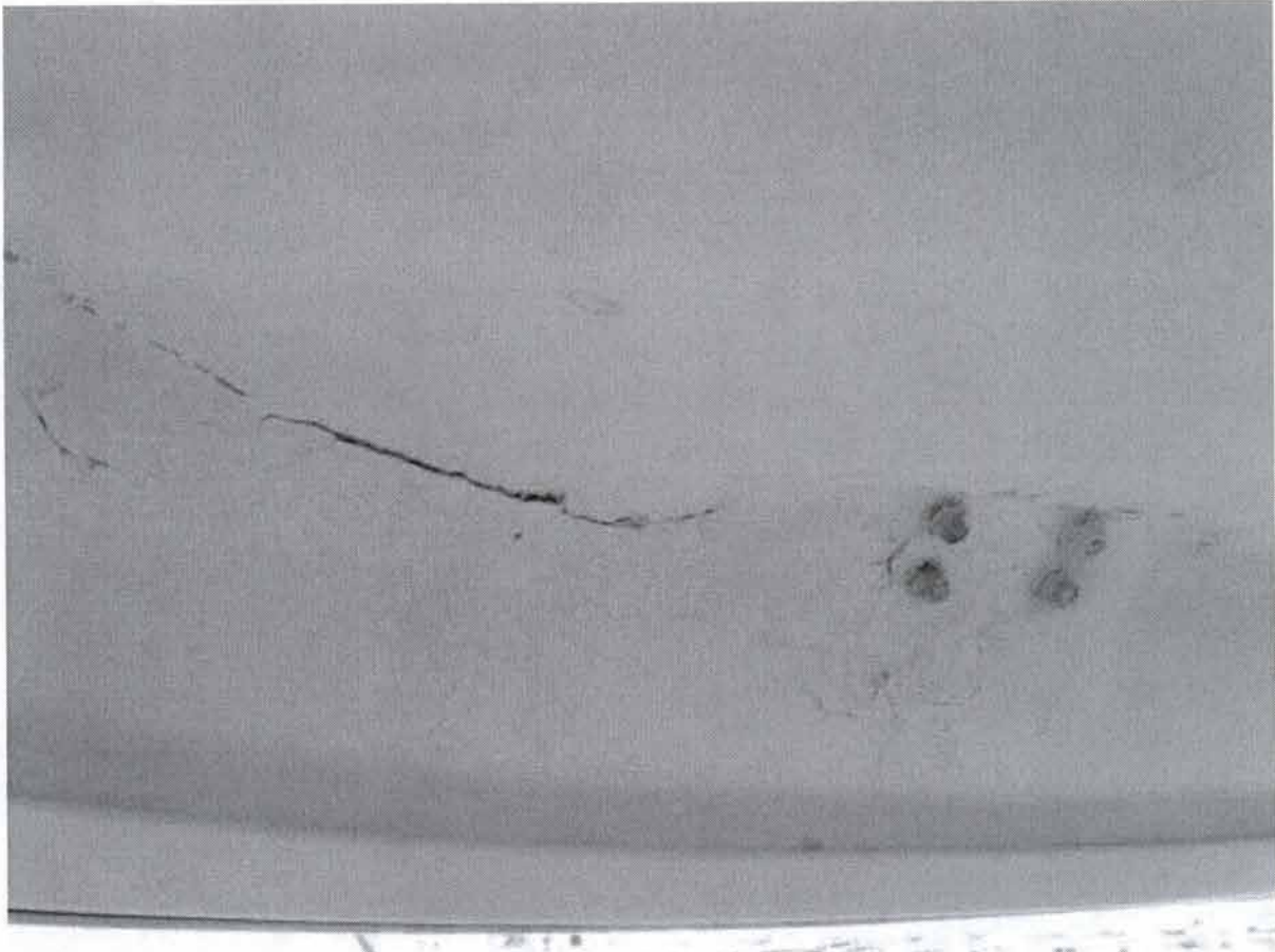
Port side underneath fresh crack
