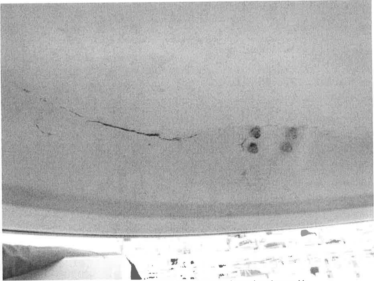
Fresh crack found underneath the swim platform associated with the exterior crack on the port side
