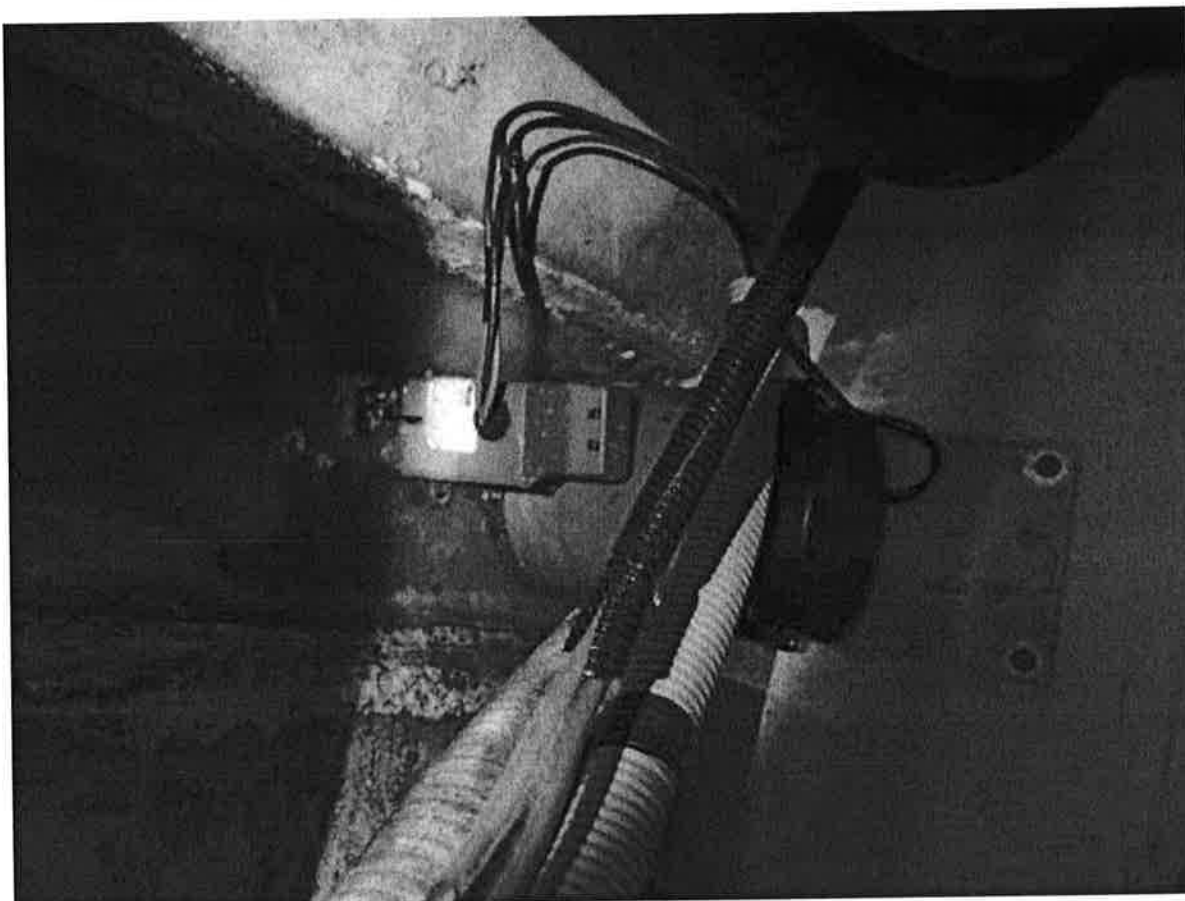
Fwd bilge pump properly wired
