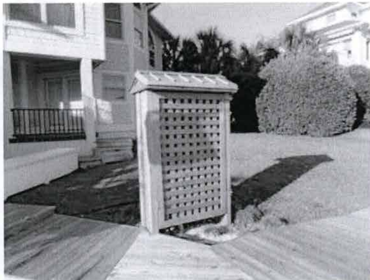
New exterior wood enclosure
